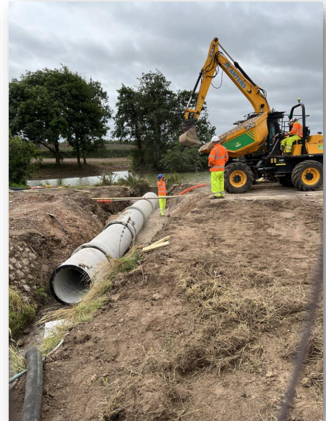
Upstream storage construction, Breedon
